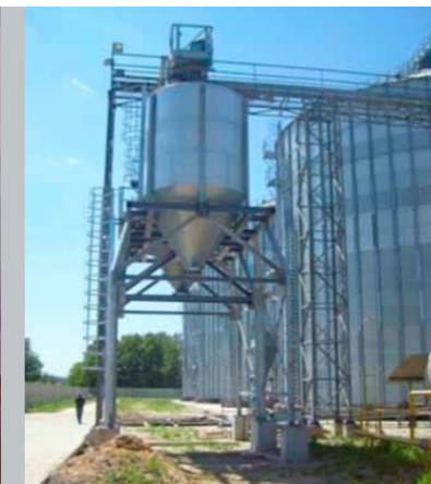
TRUCK LOADING SILOS
