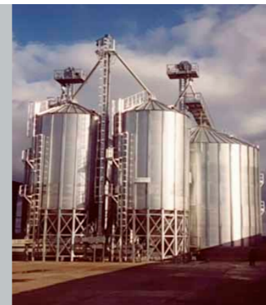
HOPPER SILOS WITH CONES OF 45^\circ & 60^\circ
